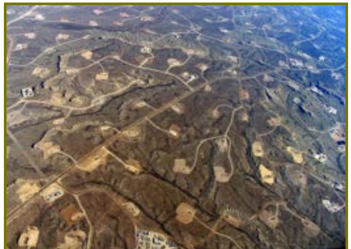
In areas where shale-drilling/hydraulic fracturing is heavy, a dense web of roads, pipelines and well pads can fragment contiguous forests and grasslands. Bruce Gordon at EcoFlight
